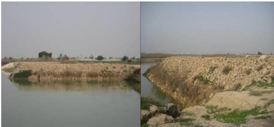
Figure 7. The spur built on Shoteyt River
